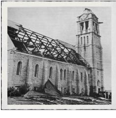
In August 1965, a tornado struck Lockport. The tornado peeled off much of the roof of the church and ripped off the taller part of the church tower destroying the statue of the Sacred Heart. Once again, Saint Dennis was repaired and rebuilt, strengthening our structure and community.
